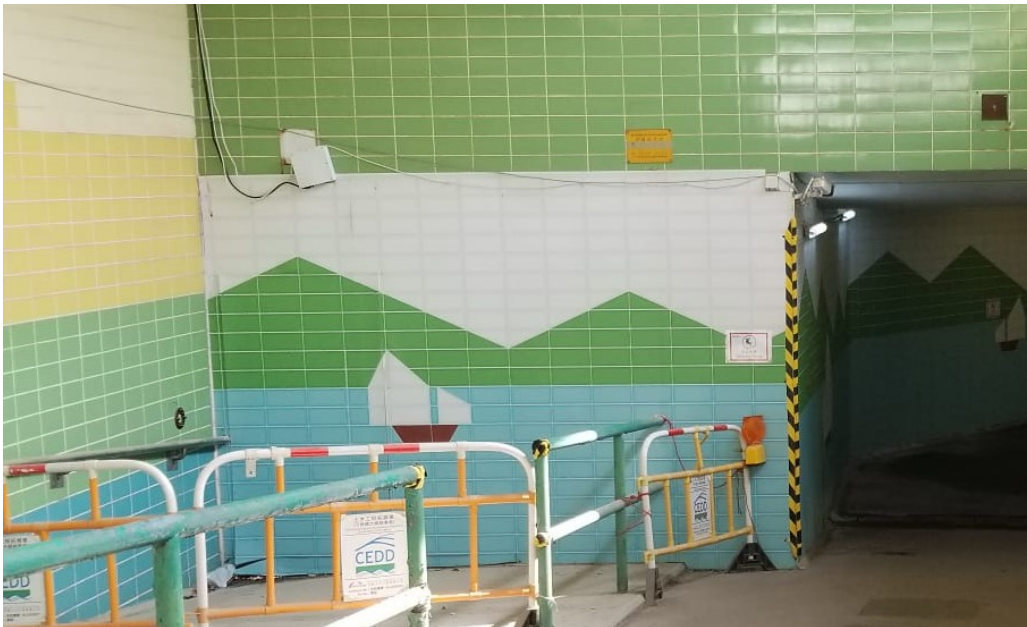
Photo 3 – Erection of site hoardings in unobtrusive colours
